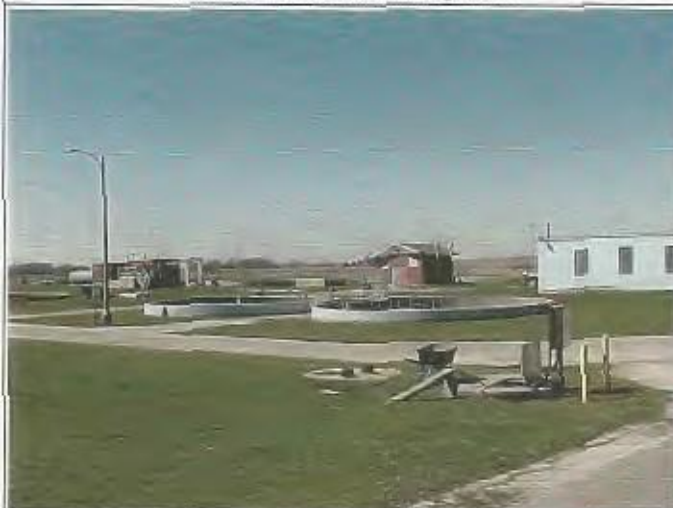
Photo 11 – Overview of Lowell Wastewater Treatment Plant.
