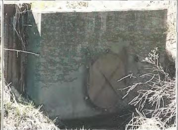
Photo 16 – CSO 004 headwall and flapgate.
