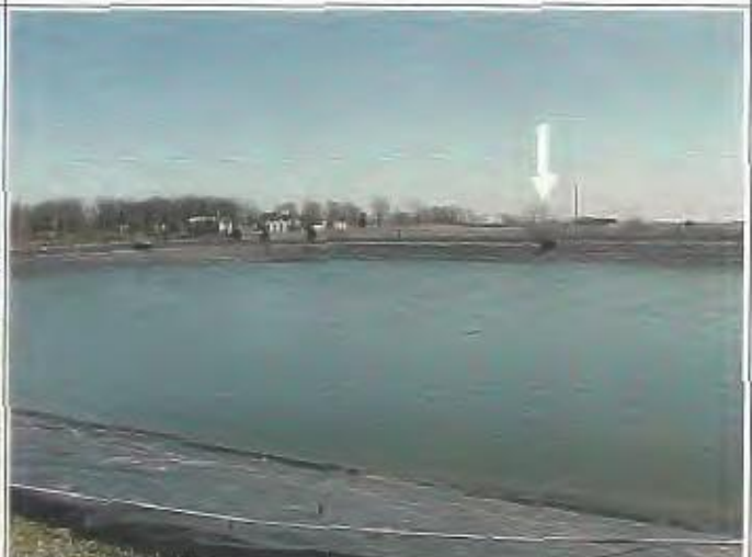
Photo 12 – CSO 007 – Stormwater equalization basin located at the Lowell Wastewater Treatment Plant. Arrow indicates the location of the CSO 004 overflow pipe.
