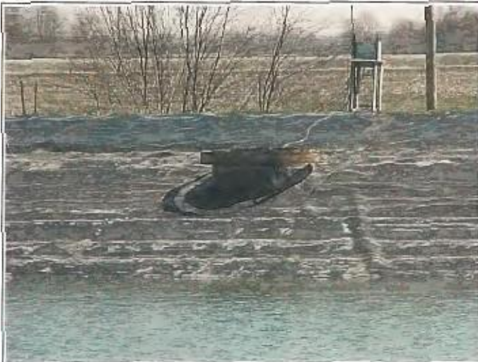
Photo 13 – CSO 004 overflow pipe from equalization basin. Basin provides floatable and solids control.
