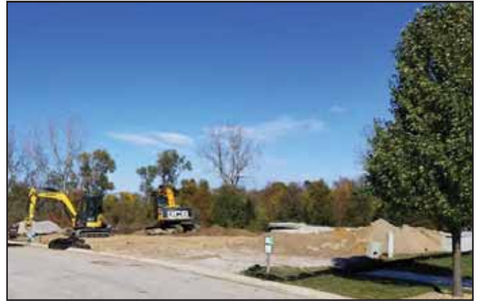
Photo 16: Overview photograph of home construction in progress. Facing north-northeast.
