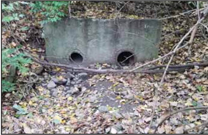
Photo 35: Photo Station 3 Facing North toward culvert outlet
