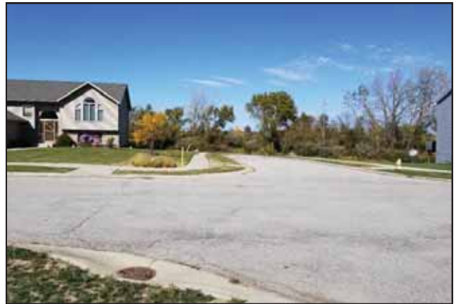
Photo 2: Overview photograph of the north end of the Project Area. Facing north from W 174 Avenue/Redbud Lane.
