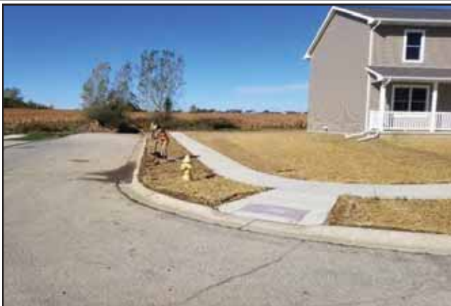
Photo 5: Overview photograph of the north end of the Project Area. Facing west from Redbud Lane.
