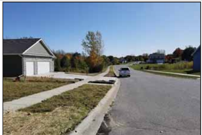
Photo 6: Overview photograph of the north-central portion of the Project Area. Facing south along Redbud Lane.
