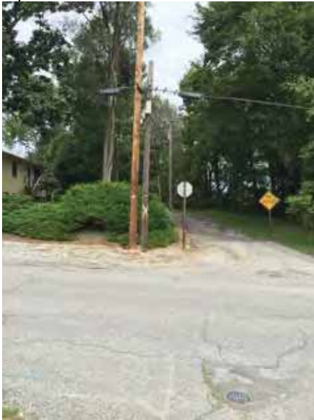
View is obstructed by power line that was replaced but not removed. There is also a large rut where a gas line was repaired and the road not restored.
