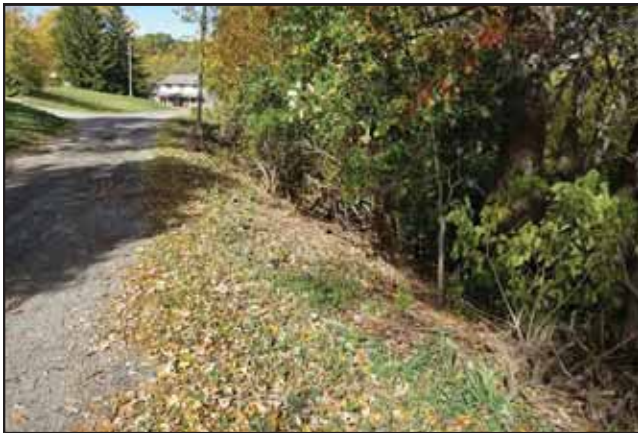
Photo 13: Overview photograph of the south end of the Project Area exhibiting slope greater than 20 percent. Facing north along N Liberty Street.
