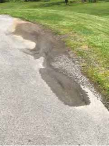
363 parking pad after water main break
